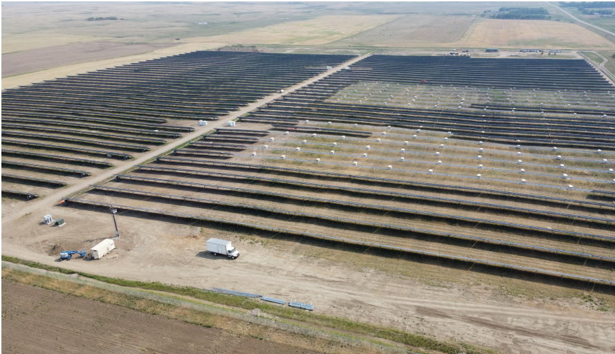
Photo of the progressing construction of the Highfield Solar Project, July 2021. Photo Credit, Ryan Hornung
